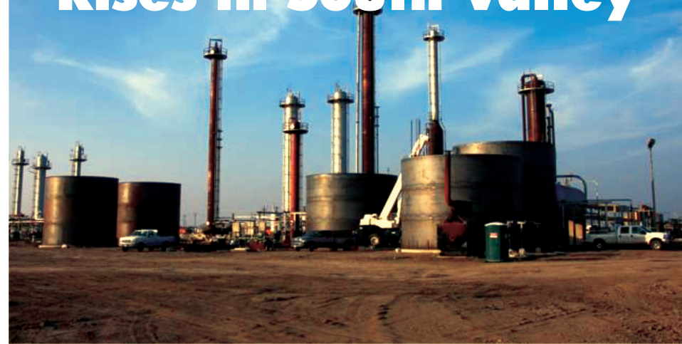
Biodiesel Plant under construction near Bakersfield.
